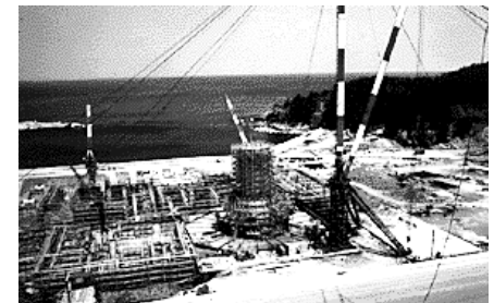
“Shimane” Unit 1 (At the time under Construction)
