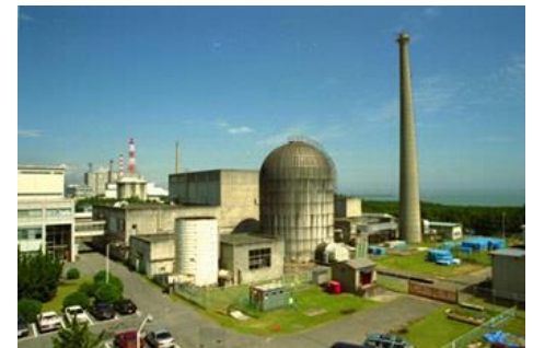
“Japan Power Demonstration Reactor” (BWR provided by GE, operated for 1963-1976)
