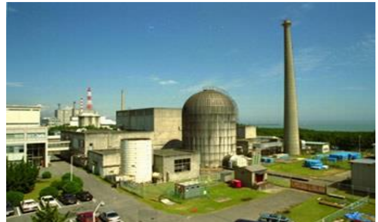
JPDR or Japan Power Demonstration Reactor (operated for 1963-1976)
