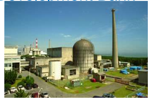
“Japan Power Demonstration Reactor” (BWR provided by GE, operated for 1963-1976)
