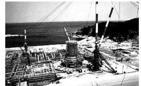
“Shimane” Unit 1 (At the time under Construction)
