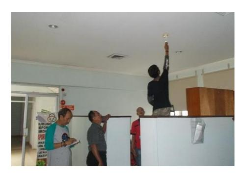
Gambar 3.17: Uji fungsi fire alaram, heat dan smoke detector
