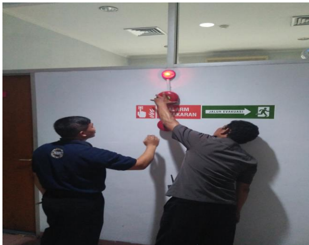
Gambar 21: Pengecekan Fire Alarm
