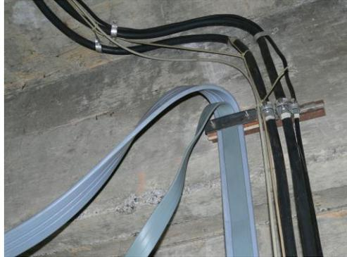
Gambar 2. Model *traveling cables*
