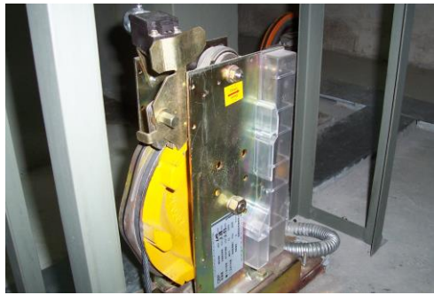
Gbr 6: Sist. keselamatan pd. Speed governor
