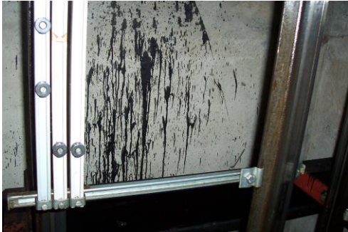
Gbr 4: Sist. keselamatan pd hoistway
