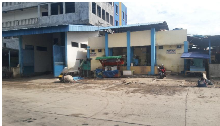
Figure 2. Toilet at Muara Angke Fish Market Source: Researcher's Analysis, 2022
