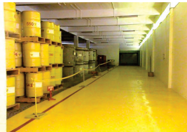
FIGURE 1. View of waste packages in IS-1 building
