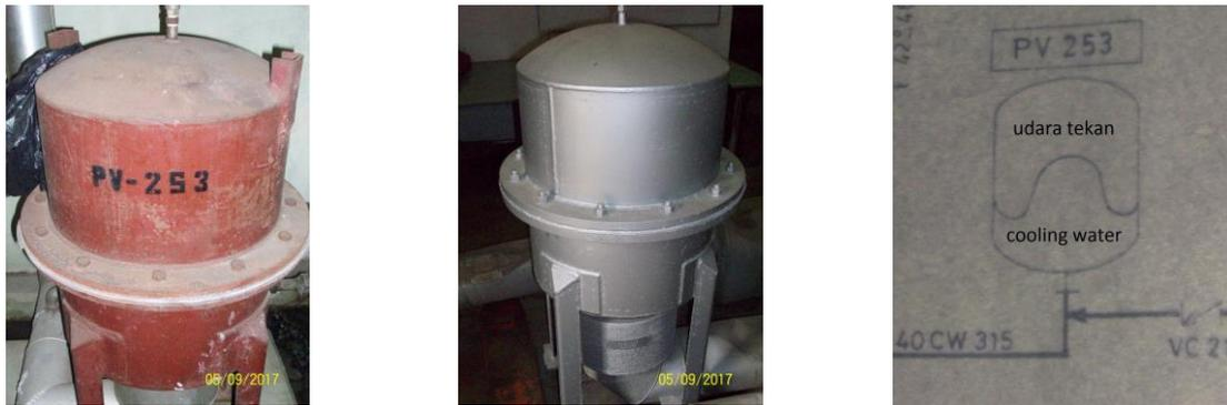
Gambar 12. Penampung air pendingin (*cooling water*), *pressure vessel type membrane*
