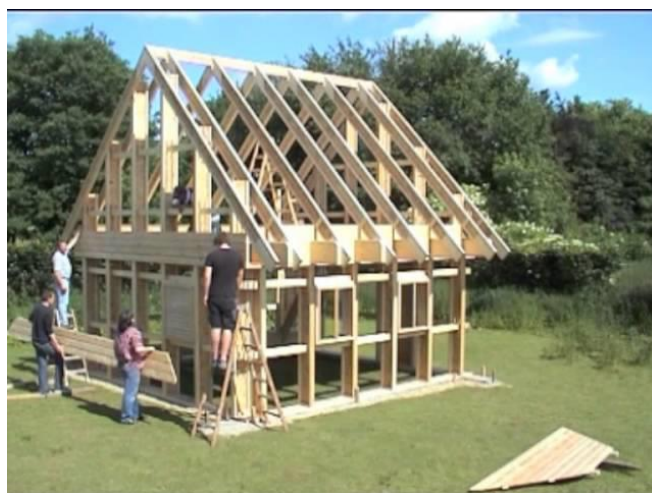
Gambar 6. Proses Perakitan Rumah Si Modular (Sumber : https://www.youtube.com/watch?v=O9myAxc3LuM )
