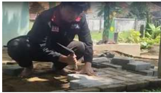
Gambar 6. Proses pemasangan paving block
