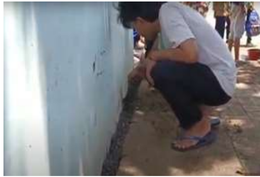
Gambar 8. Proses penguncian paving block
