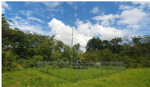
Gambar 2. Kondisi Menara Base Transceiver Station (BTS) di Kampung Baingkete
