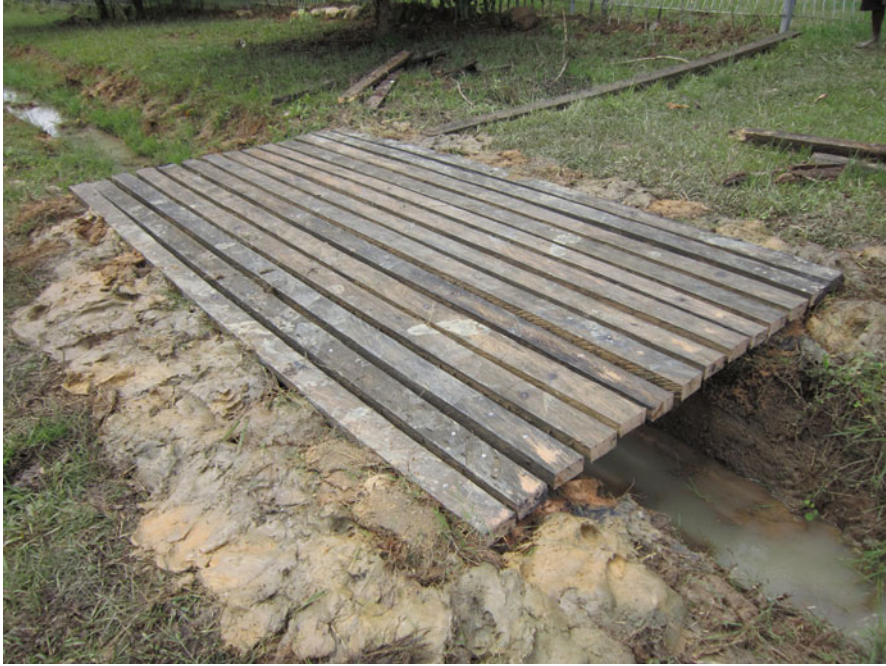
Fig. 3 Wood used in bridge construction. (© Ary P. Keim)
