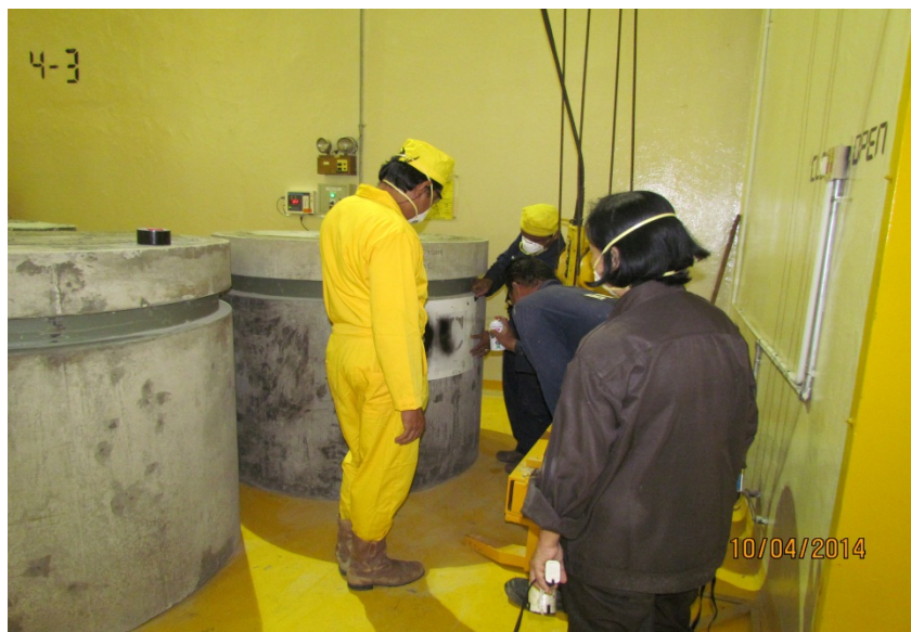
Gambar 1. Proses penomoran Shell beton
