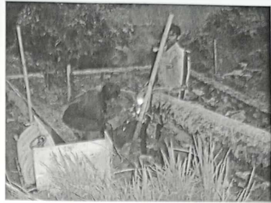
Pengelasan pipa penstock
