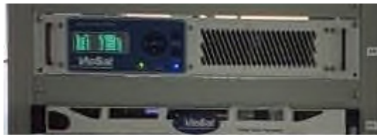
Gambar 2.3 Modem VHR (ViaSat High-Rate Receiver ) 1200 dan Modem VDP (ViaSat Data Processor) yang terpasang di ruang server
