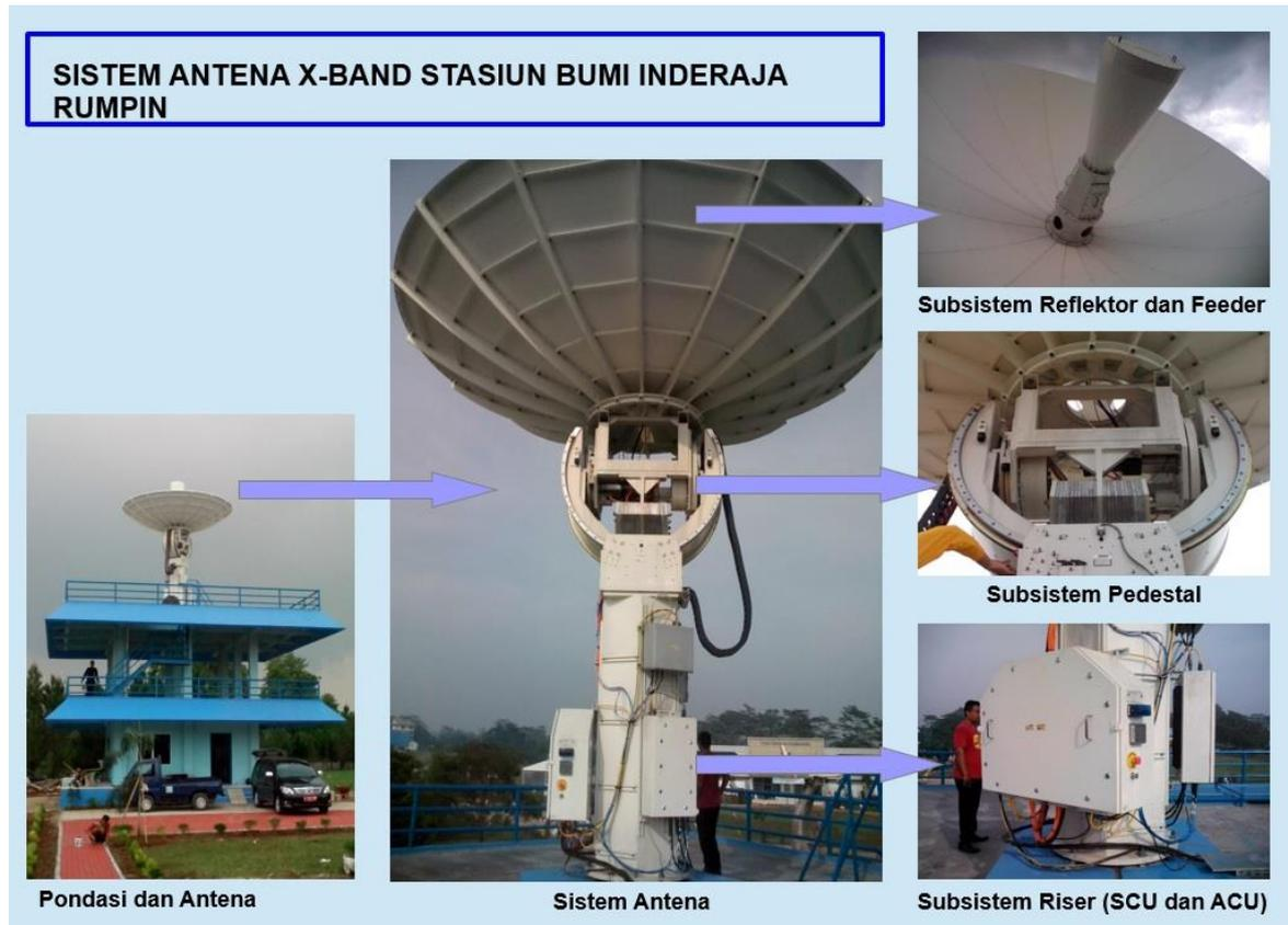
**Gambar 4.** Sistem eksisting antens X-Band 5.4 m Viasat
