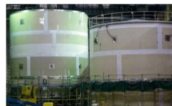
RWST is being fabricated at facility
