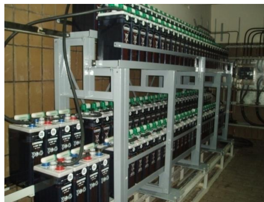
Gambar 3. Susunan batere BT03 (type 4 OSP.XC.160)
