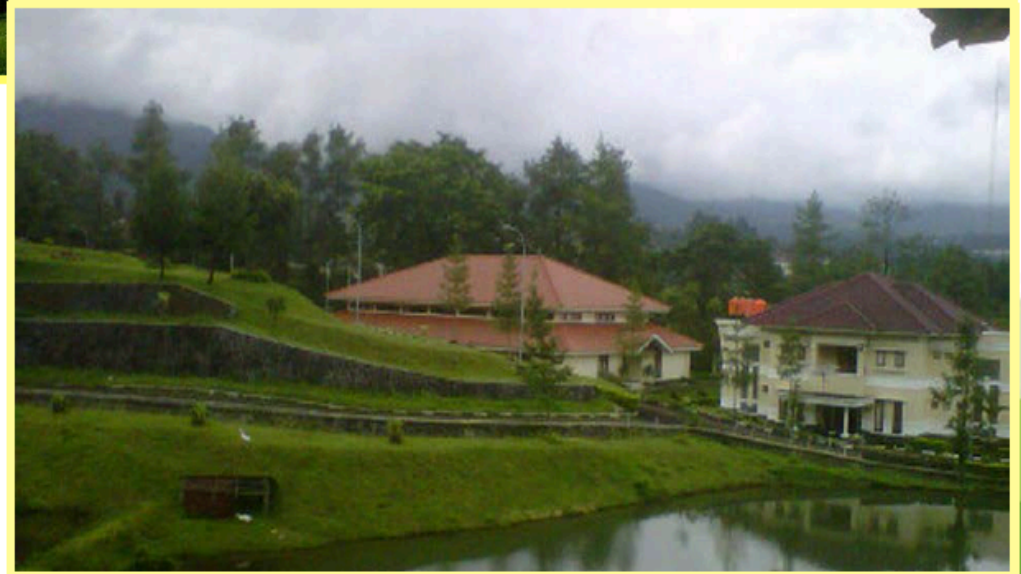
BAPETEN Education and Training Facility (Badiklat) Cisarua – Jawa Barat
