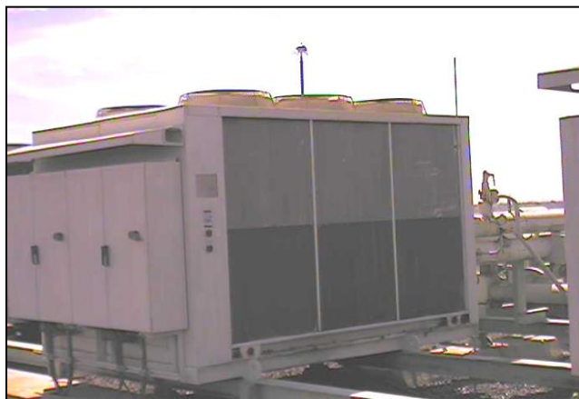
Gambar 3. Chiller water system, CWU; QKJ10/20/30 RSG-GAS [3]
