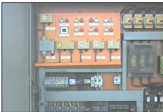
Gambar 5. Hasil scanning panel chiller water system , CWU; QKJ20 RSG-GAS
