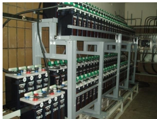
Gambar 3. Susunan batere BT03 (type 4 OSP.XC.160)
