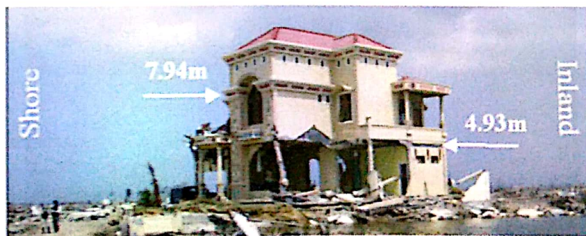
Fig. 9. Partially damaged family house located about 0.9 km inland in Banda Aceh. Left side is shore and right side inland. Numerals indicate inundation depths
