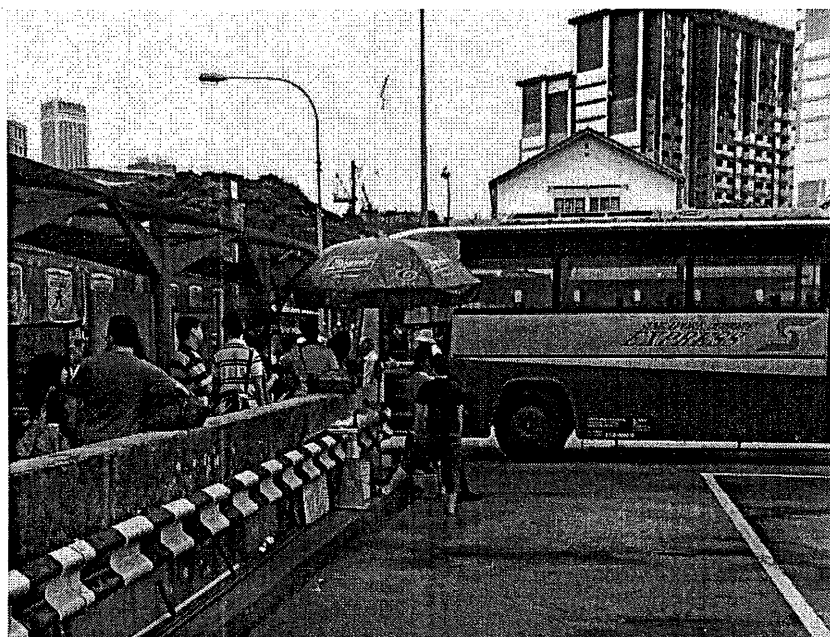
Plate 4.2. Bus terminal in Singapore
