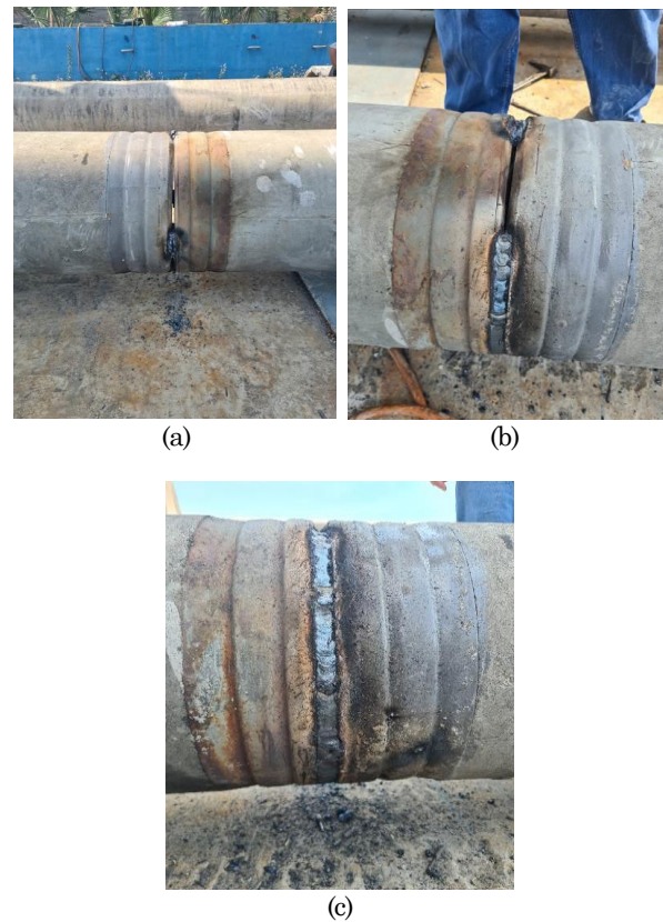
Figure 7. (a) Welding at Four Points; (b) Welding at Half Circle; (c) Welding Full Circle
