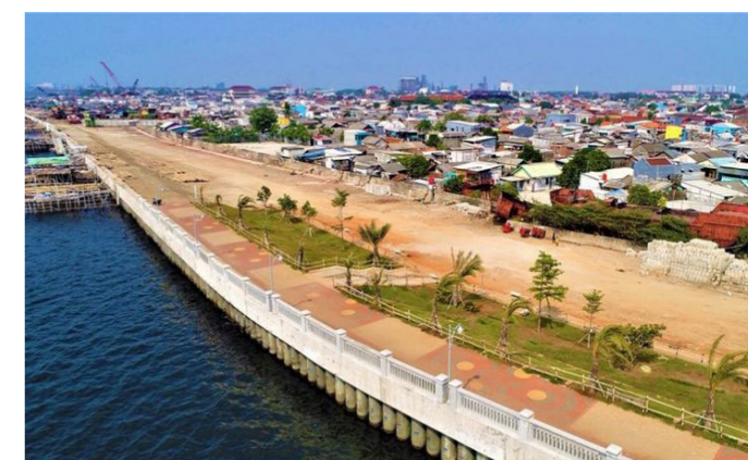
Sea Wall in Muara Baru, North Jakarta (Kemen PUPR, 2019).
