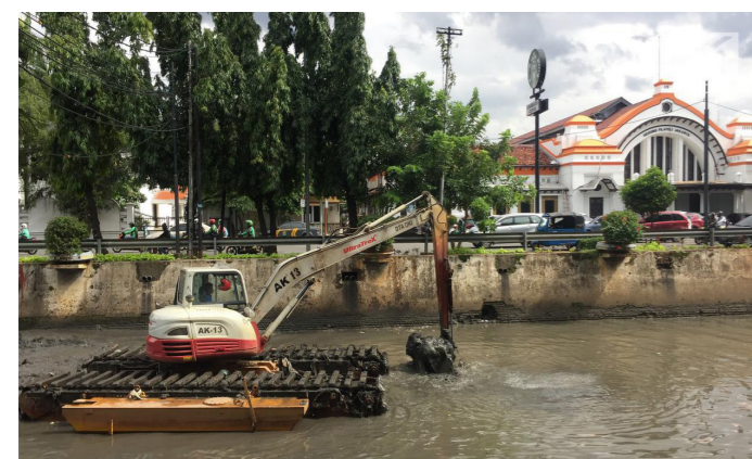
River dredging in Sawah Besar, Central Jakarta (Liputan 6, 2020).
